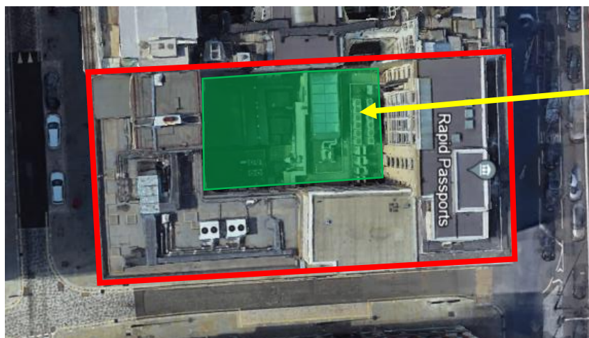
Initial demolition for Tower Crane enabling works and installation
