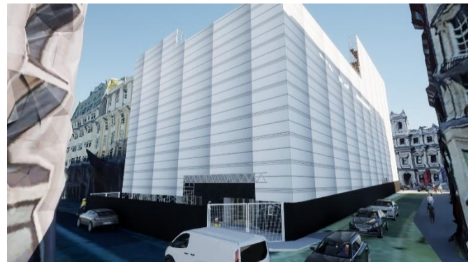
Hoarding, scaffold and pit lane arrangement Duke St and Jermyn St
