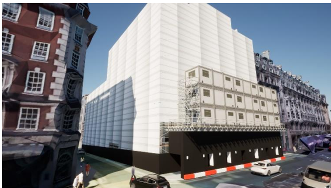
Hoarding and scaffold arrangement Piccadilly Rd and Duke St
