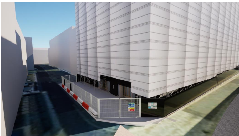
Hoarding, scaffold and pit lane arrangement Duke St and Jermyn St
